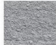
CSP 4 (light scarification)
