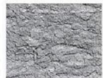
CSP 6 (medium scarification)
