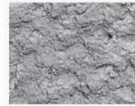
CSP 7 (heavy abrasive blast)
